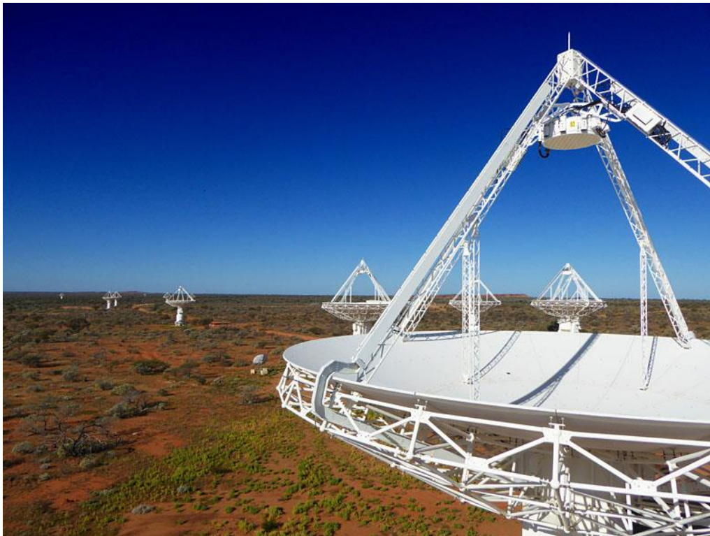
The ASKAP radio telescope with its innovative phased array feed receives (at apex of antennas). Photo credit: CSIRO
